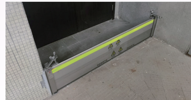
Flood Gate at Regal Airport Hotel
