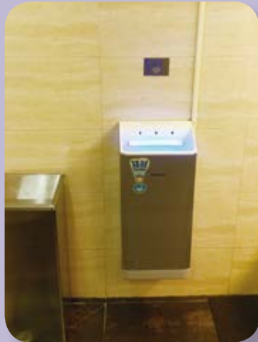
Installation of hand dryers in washrooms
